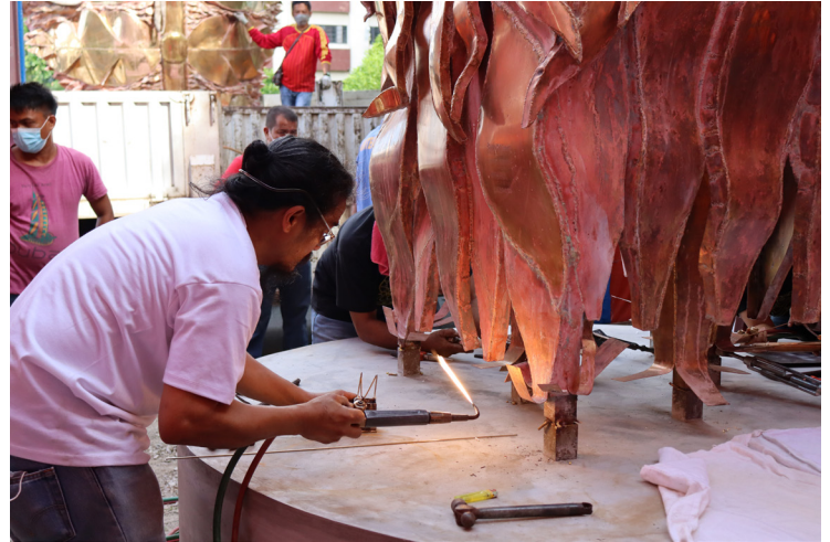
^ Villanueva welds the base of the sculpture, cementing his mark in UMak’s history.
